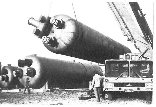
Electric separators for removing the water from the oil being hoisted and installed.
