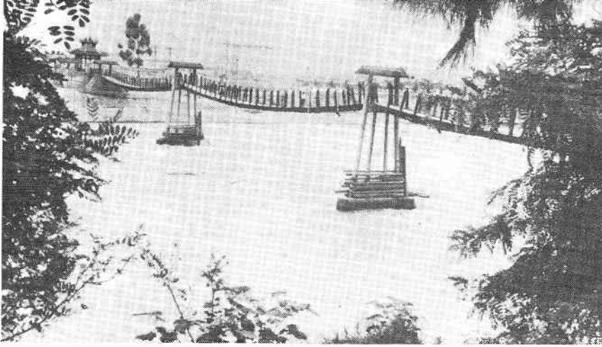
The half-kilometer suspension bridge spanning the dividing of the waters at the ancient Dujiangyan irrigation project.
