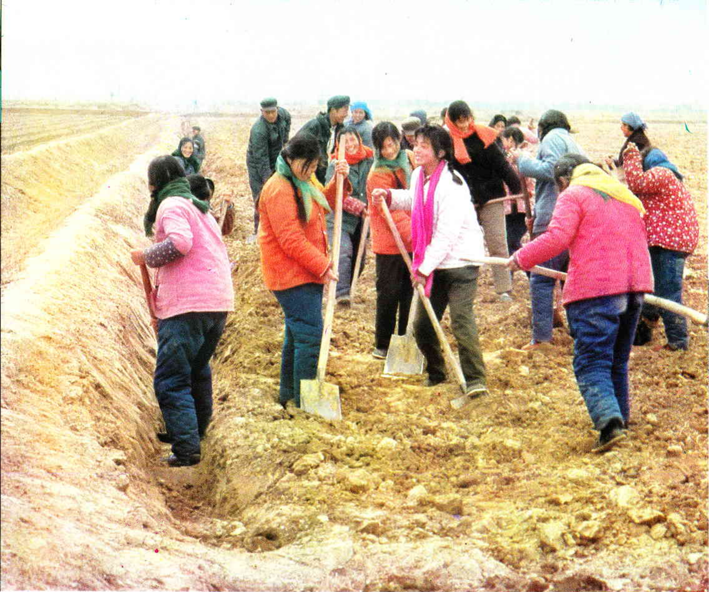
Building a canal.
