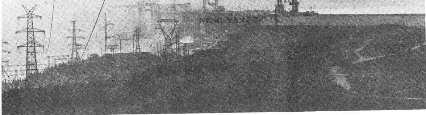
The Danjiangkou in Hubei province, one of China's biggest water control projects, generated record amounts of electricity during last year's flood.
