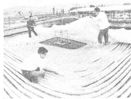
Pipe for solar heated water made from plastic film at the Yunnan Institute of Architectural Science. Zhou Zhongyao
