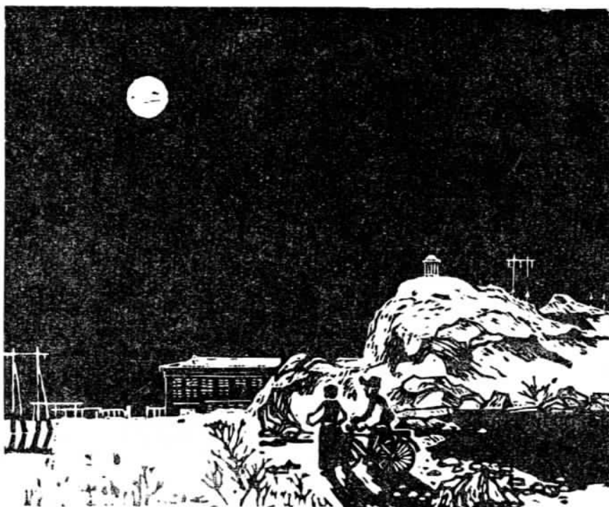
Hydro-Electric Station in Tibet
