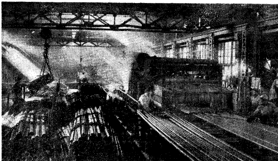
Workshop in the Shanghai Irregular-Shaped Steel Tubing Plant
