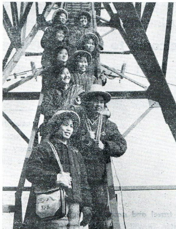
Installers of the Wuhan Power Supply Bureau.
