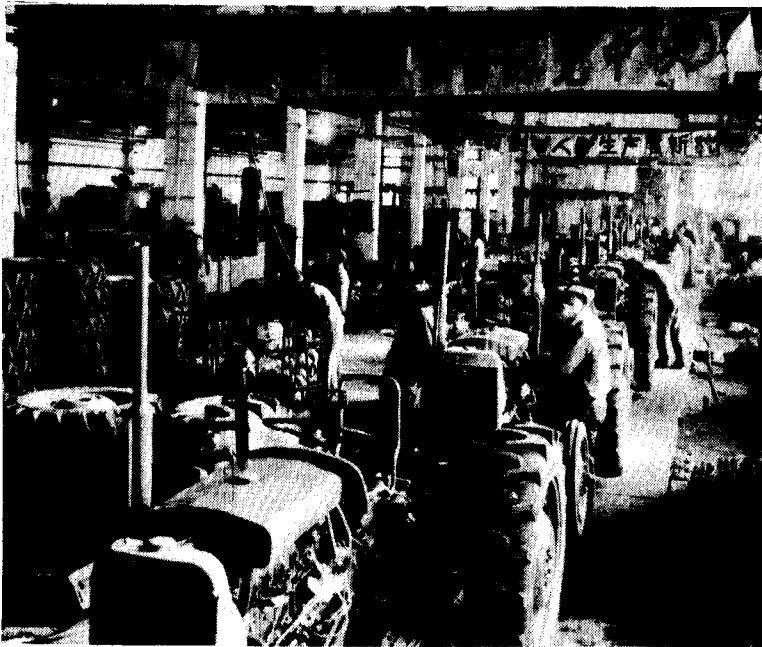
The plant is now in full operation.
