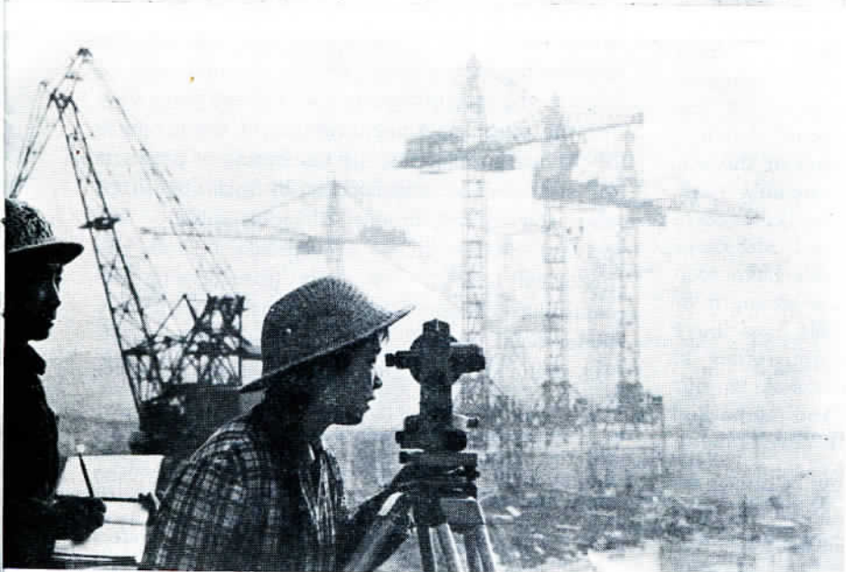
Building the giant Gezhouba Hydropower Station on the Changjiang River.
