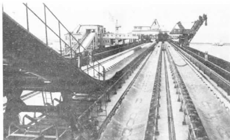
A new landing stage at Qinhuangdao coal dock, Hebei Province.
