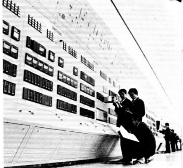
Workers at the Shanghai Petrochemical Complex installing instruments and meters.
