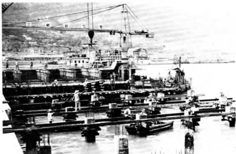
Construction to expand Lianyungang Port in Jiangsu is under way.
