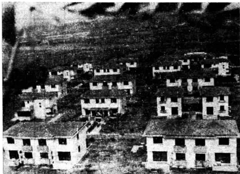
Newly built houses for foreign oil co-operative partners in Zhanjiang.
