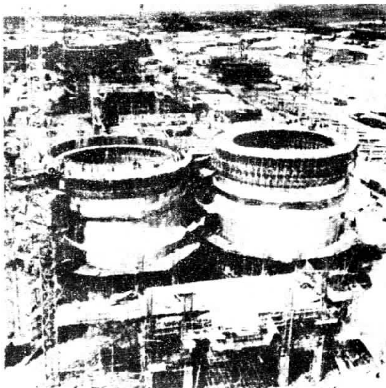
Construction of the Ninggou Cement Plant in Anhui.
