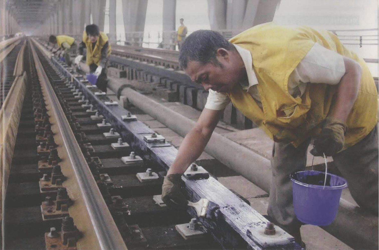
RAILWAY SAFETY: Workers at the Jinan Railway Bureau grease the tracks
