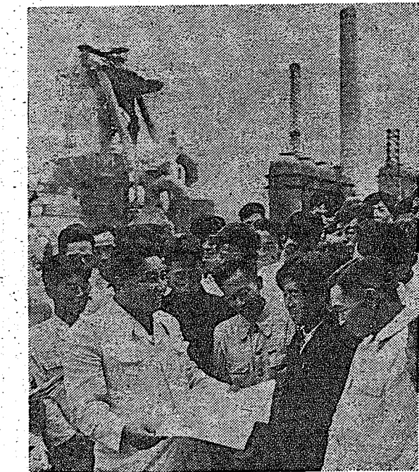
KPDR Premier Kim Il Sung in the Wanghai Iron Works.
