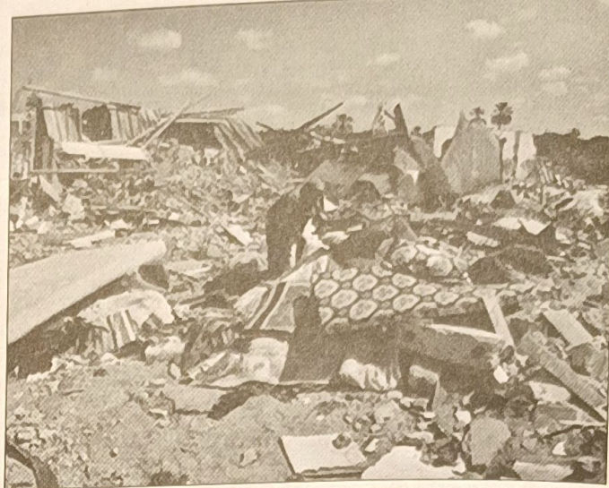
House in Gaza destroyed by Israeli forces, September 2007
