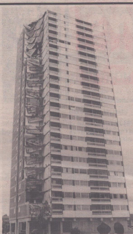
The Ronan Point tower block in London's East End after the 1968 gas explosion
