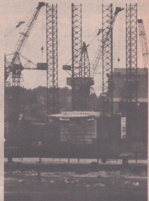
The occupied rig at Cammell Laird
