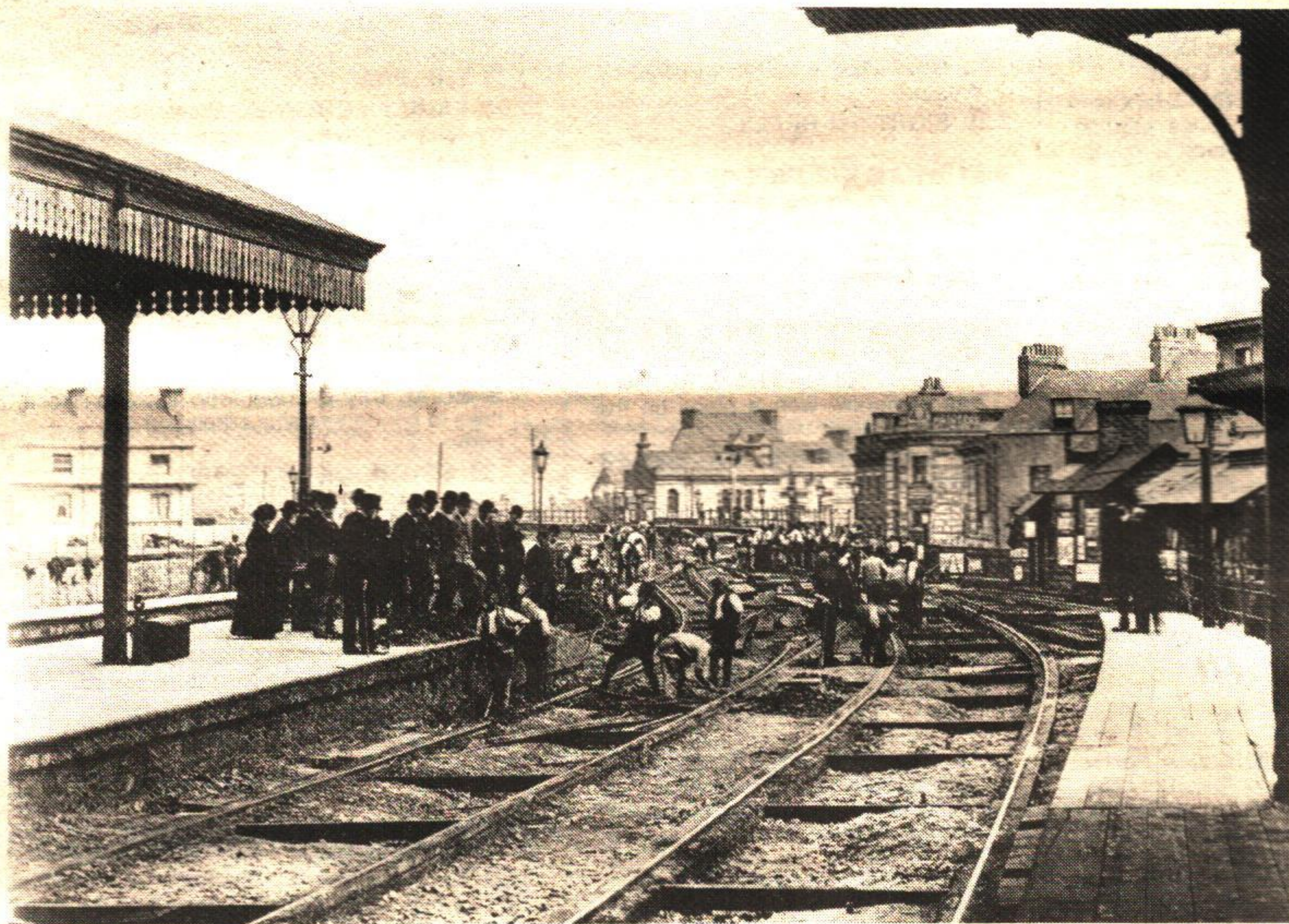
May 21st, 1892, Plymouth station: gangs of workmen replace over 400 miles of the old broad gauge with the standard 'coal-cart gauge' in a single weekend
