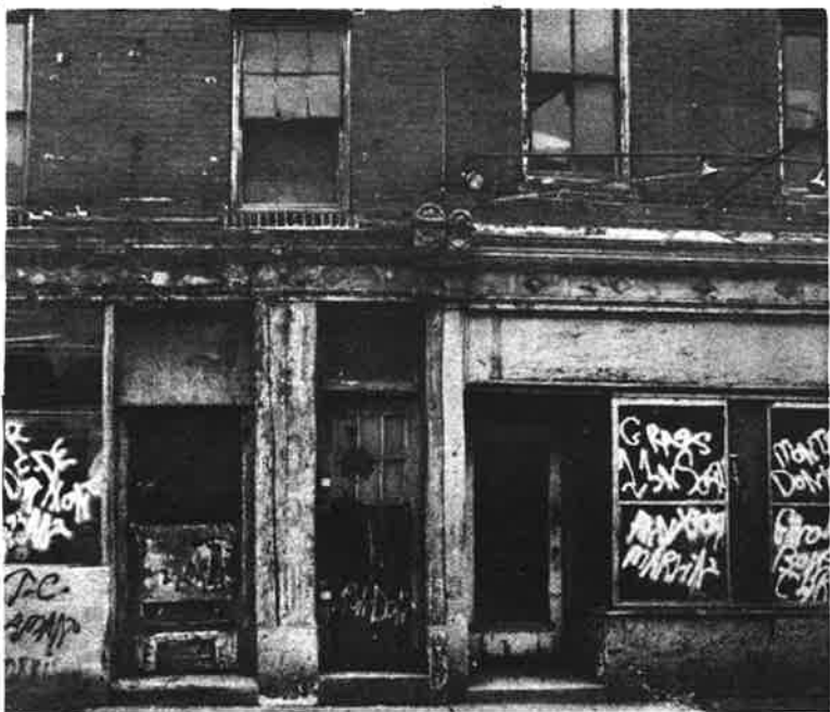
An abandoned apartment building in Philadelphia. Carter is proposing a $3.2 billion tax give-away to big business, while millions of poor people don't even have a decent place to live.
