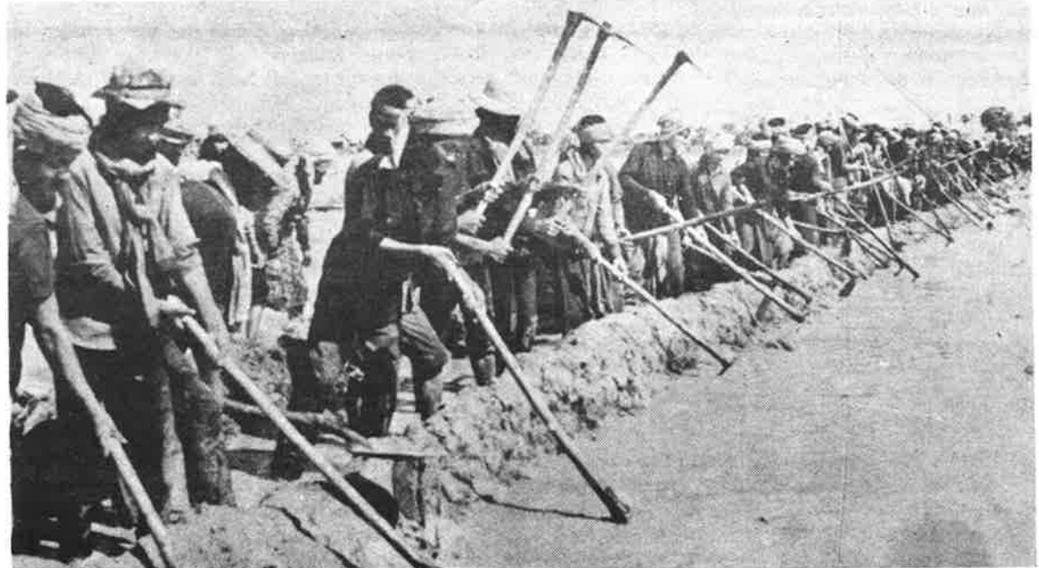
The people of socialist Kampuchea [Cambodia] work together to build irrigation canals and new embankments for rice fields.
