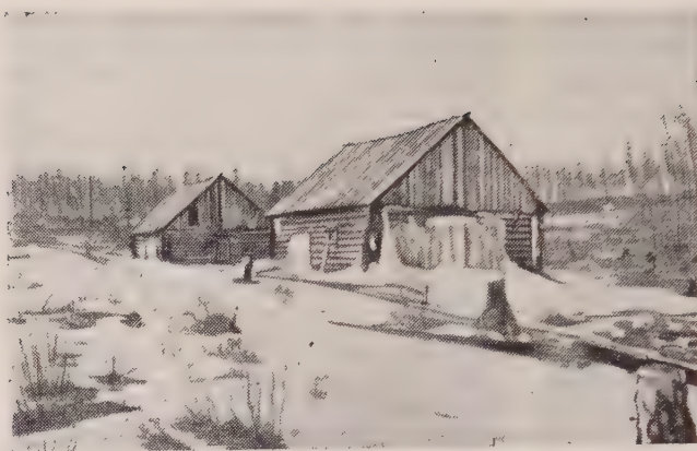
This house is built on eternally frozen ground. The ice beneath has melted, the water risen through the floor, filled the building and poured from the windows
